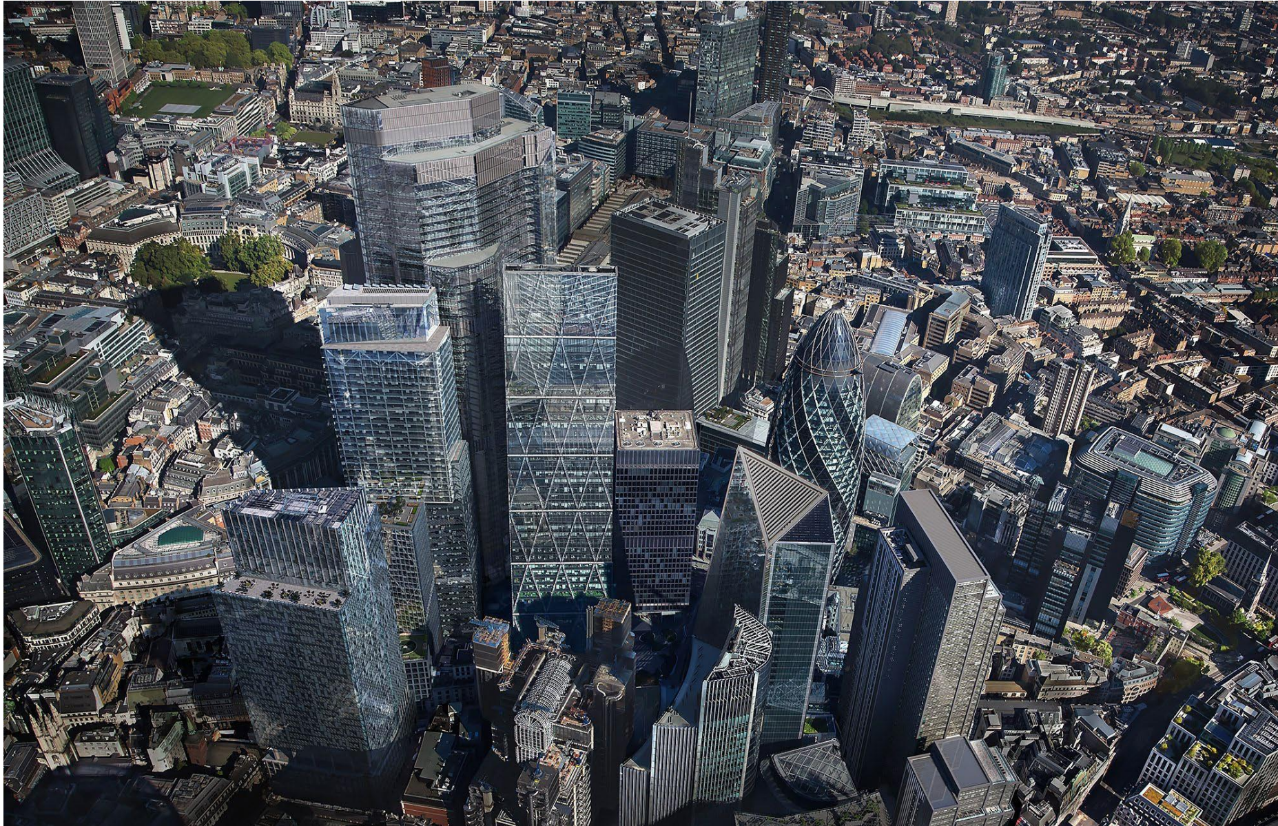
Aerial view of existing site
